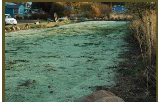
Landscaping phase 2 - in progress
