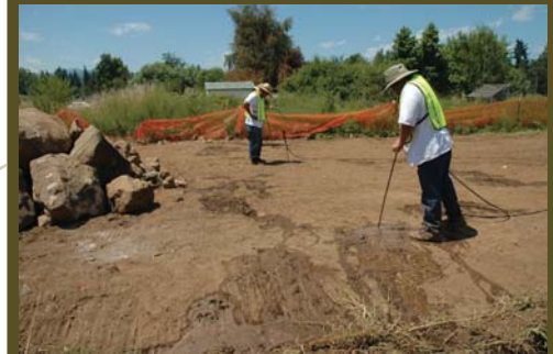
In-situ injection of GMS products
