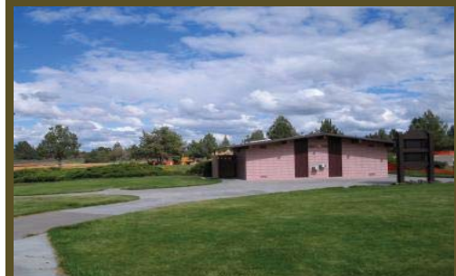
Highway rest area
